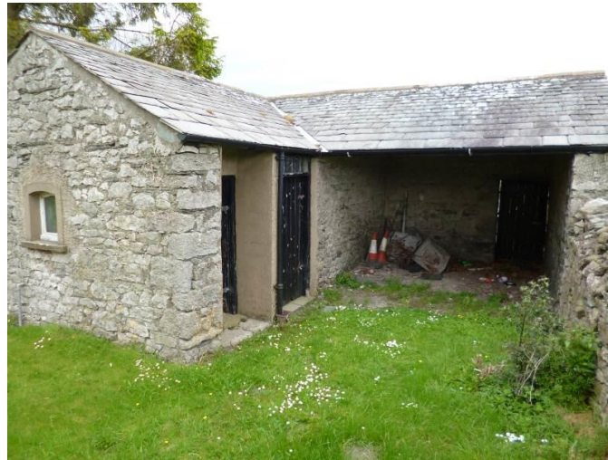
Fig.5: gig house and stables in south-corner of the grounds
